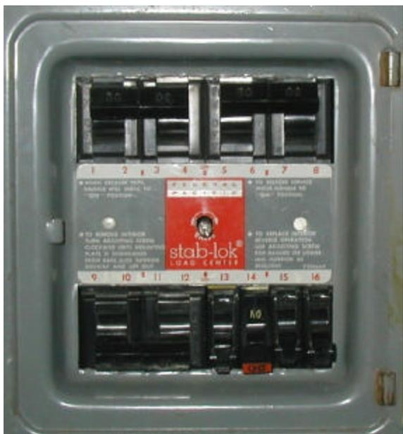
Figure 2 – Breakers that are on when down
